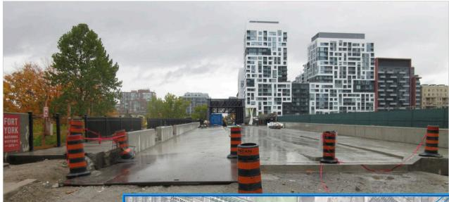
Where the Brock Bridge touches the ground at the south-east corner of Fort York. Shrouds are off the steel trusses in the distance, the roadbed has been poured and streetcar tracks are being stockpiled nearby. In the curb at left can be seen the outline of a stop for the Bathurst 511. Despite the progress, another month has been added to the project: the City is now promising completion by the end of January. Photo by the F&D
